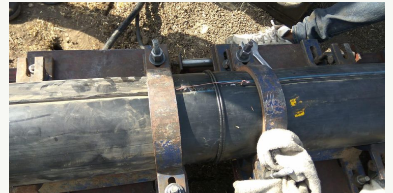
Pipe joint assembly on site
