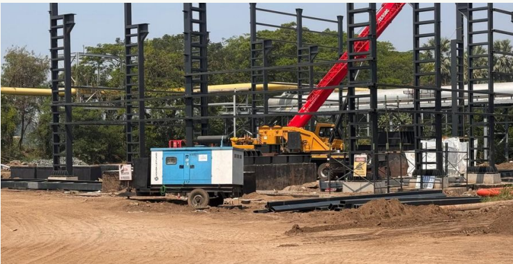
Structural erection at site
