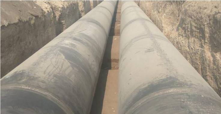
Large-diameter water pipeline in trench
