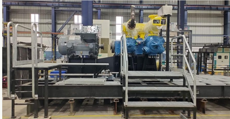
Compressor equipment erection
