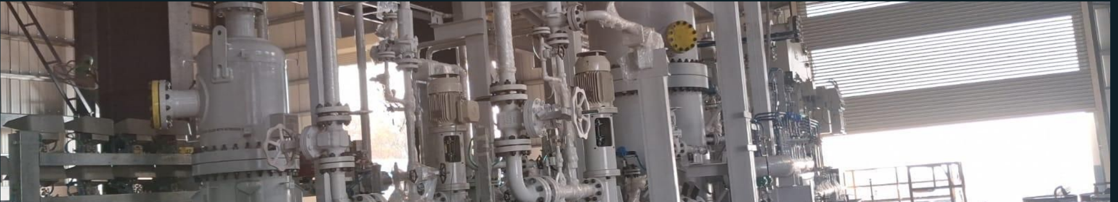
Flare-line skid under fabrication in our workshop.
