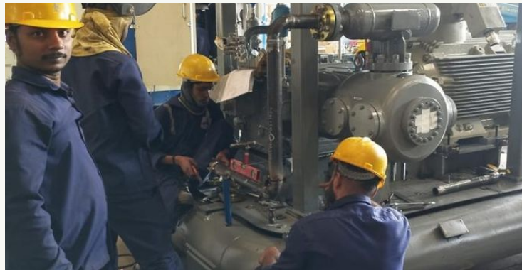
Skid fit-up in the workshop
